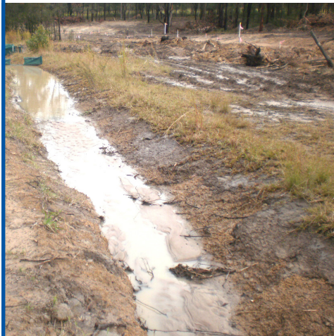
Diversion channels/catch drains/dirty water
