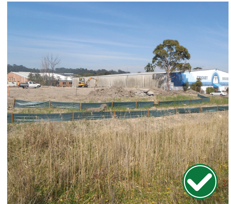
Buffer zone and sediment fences
