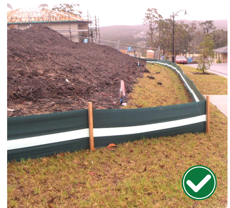
Mulch for erosion control and sediment fence for sediment control
