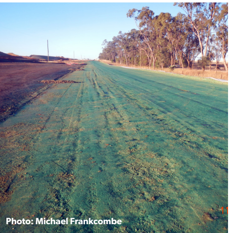
Dust control with a polymer
