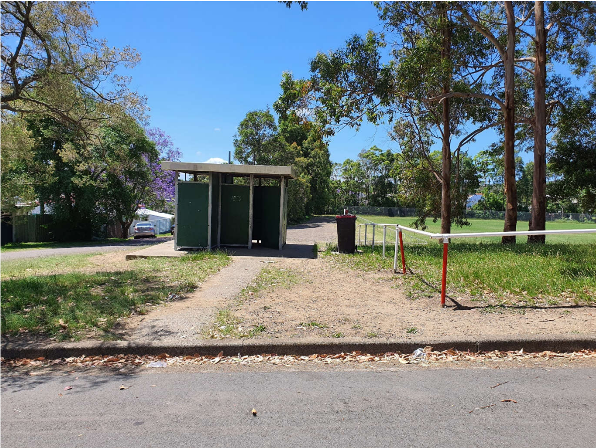
Figure 10: Review of existing facilities should include condition and suitability of the location.
