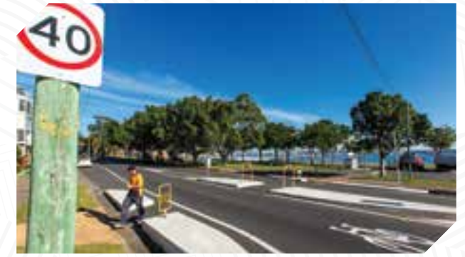
Kerb extensions and refuges to improve safety, especially for children, the elderly and people with disability
