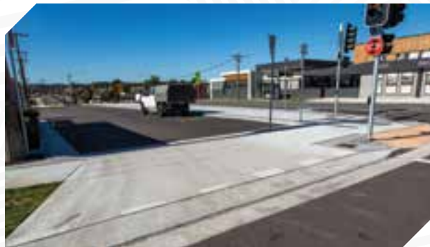
Continuous path treatment across local streets, to give pedestrians and cyclists right of way and to help reduce traffic speeds
