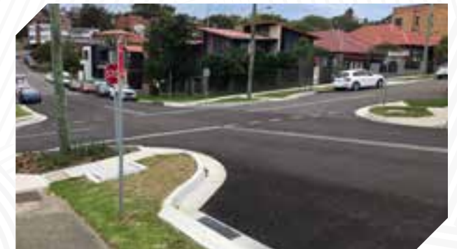
Kerb extensions and narrow intersections reduce pedestrian time spent in the roadway area
